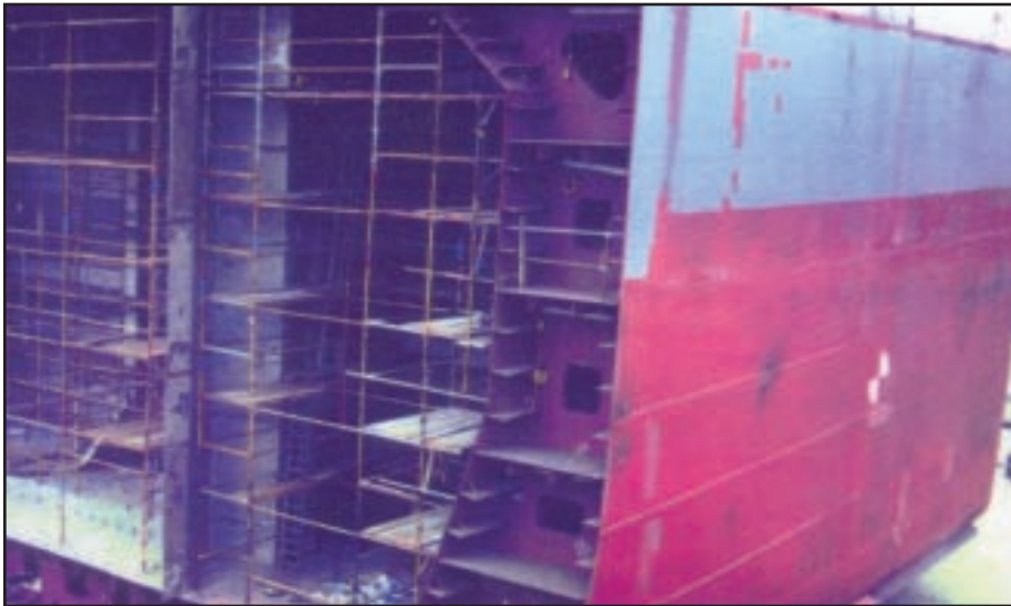
Fig 1. Large section of a ship being joined with Kat Oscillation.
