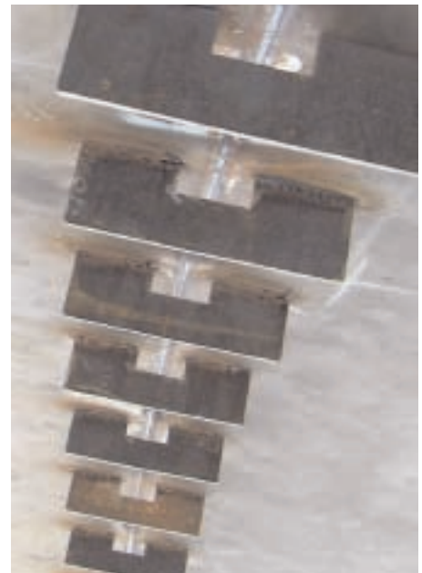
Above: Gullco KATBAK with self-adhesive tape fits through cut outs in the strong backs. The use of KATBAK in this application enabled single sided welding (below) on the outside of the sphere...resulting in the root side of the joint inside the sphere (right) being as good as the outside.
