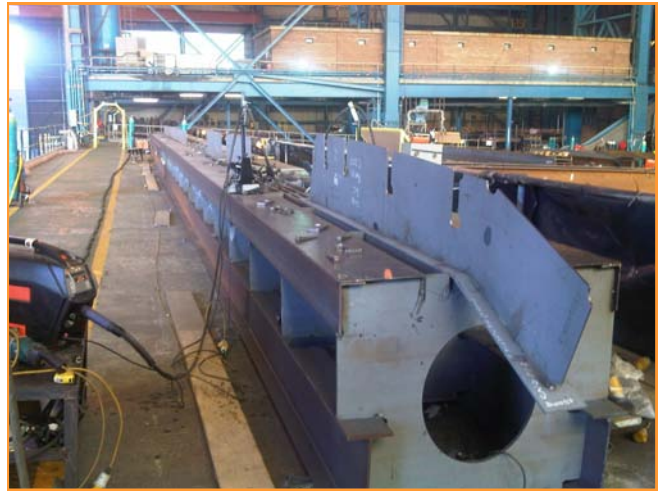
Moggy® Trackless Welding Carriage System completing structural fabrication on UK aircraft carrier.
